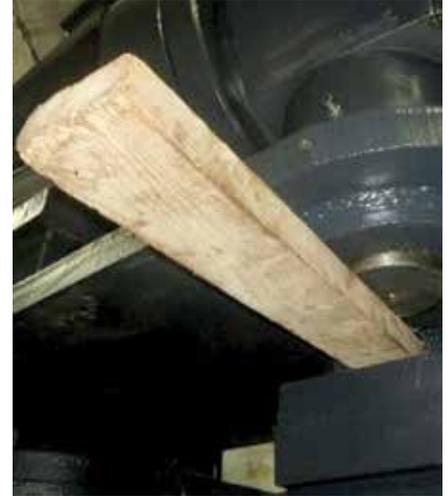
**A plank supports** emergency-closure valve pins in the Kajaki Dam Irrigation Tunnel. (SIGAR photo)
